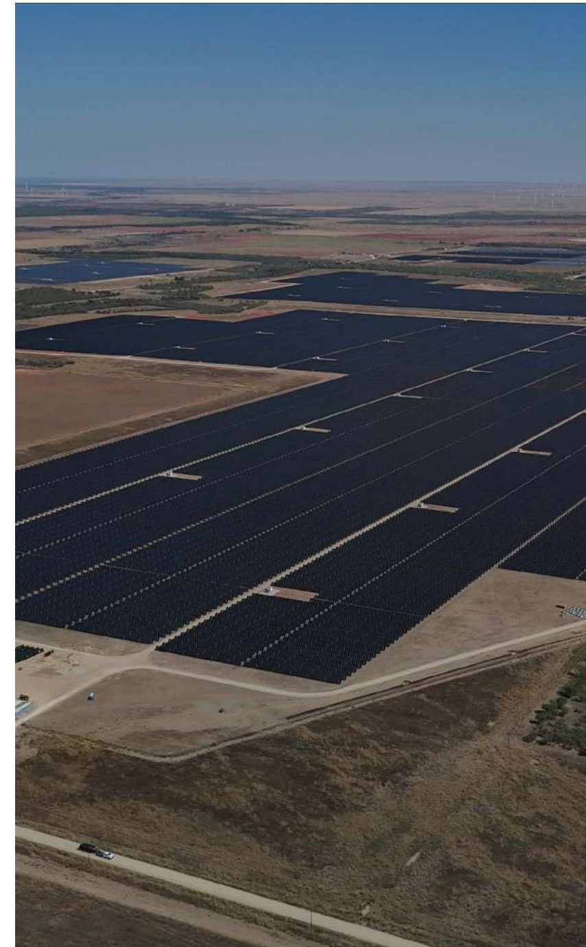
The Millers Branch Solar Facility in Haskell County, Texas (pictured right) is expected to come online in 2026.
